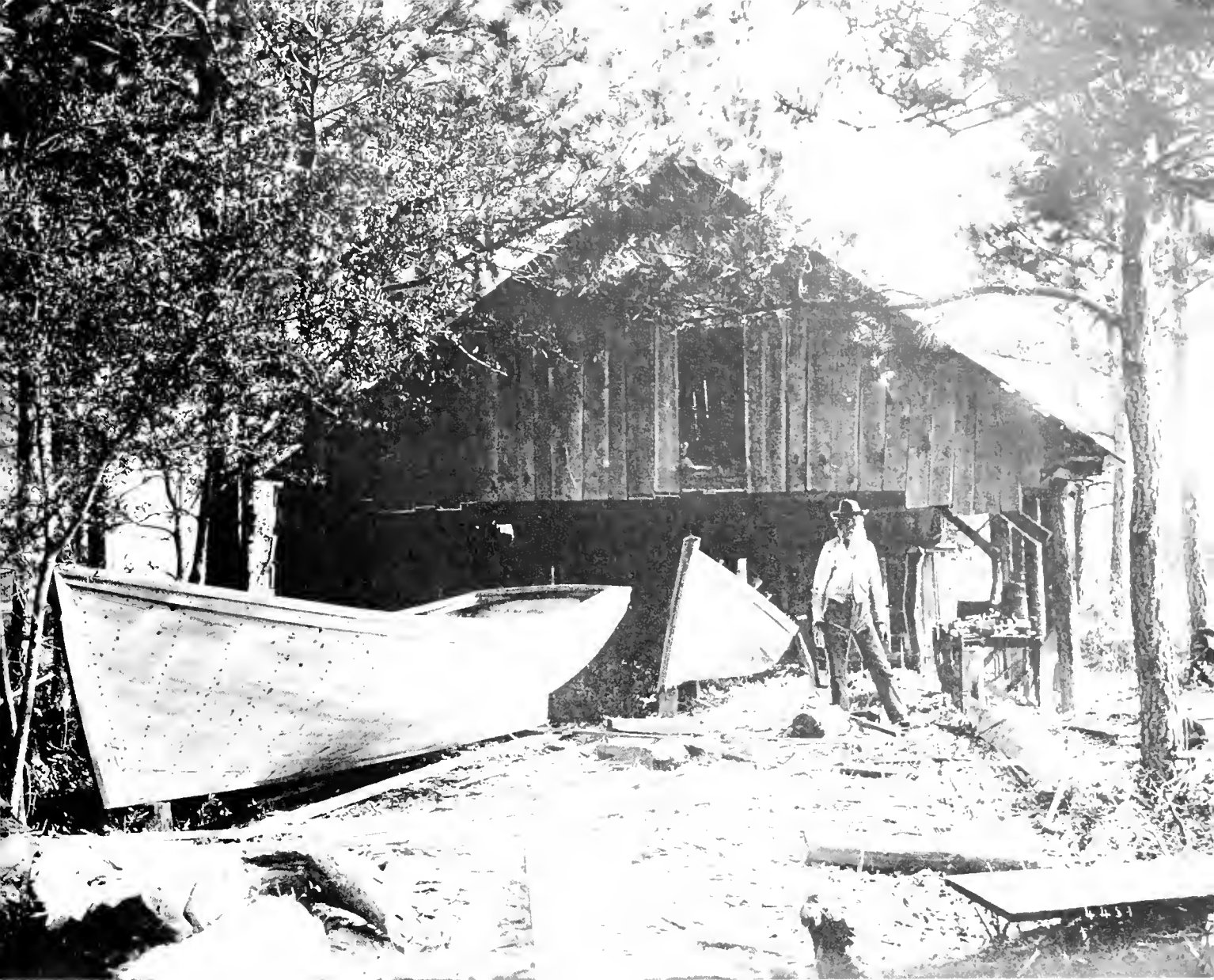
AT BERMARIE SOUND SHAD BOATS BEING BUILT AT ROANOKE ISLAND, NORTH CAROLINA, at the yard of the noted local builder, Washington Creef, in the 1890's. These boats, fitted with planked stern deadwoods, are large for their class. A good example of the simple boat shops in which these small fishing boats were built. (Smithsonian photo 44793 f.)
